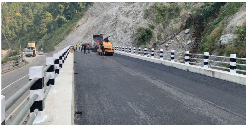
Figure 4 – Namsi Bridge, Chitwan
