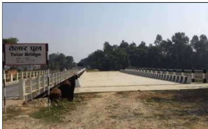
Completed Telar Bridge, Rupandehi
