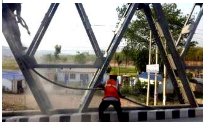
Sand Blasting work at Girwari Khola Bridge(45-H001-249)
