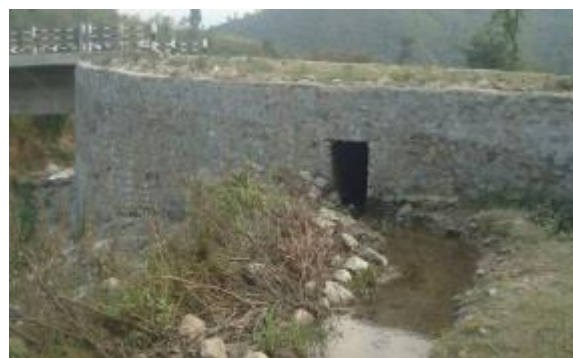
Reinstated irrigation canal, Kawa Khola Bridge
