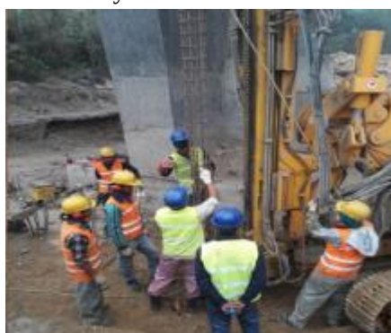
Workers on duty with safety gear
