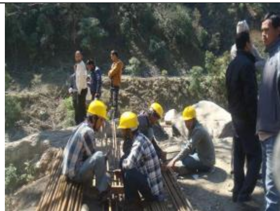
Workers on duty at Tipadagad bridge
