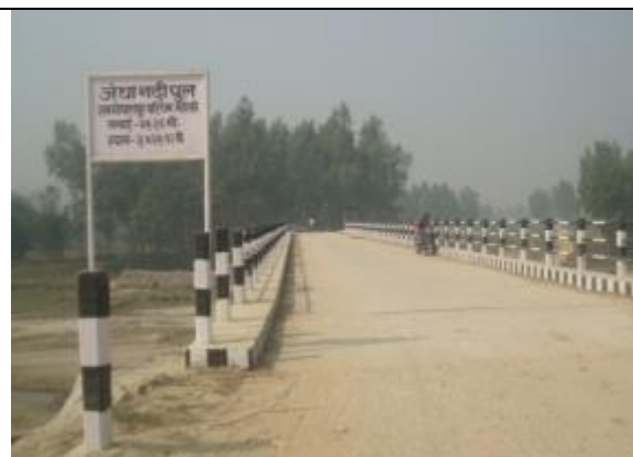
Completed bridge Jangaha river bridge
