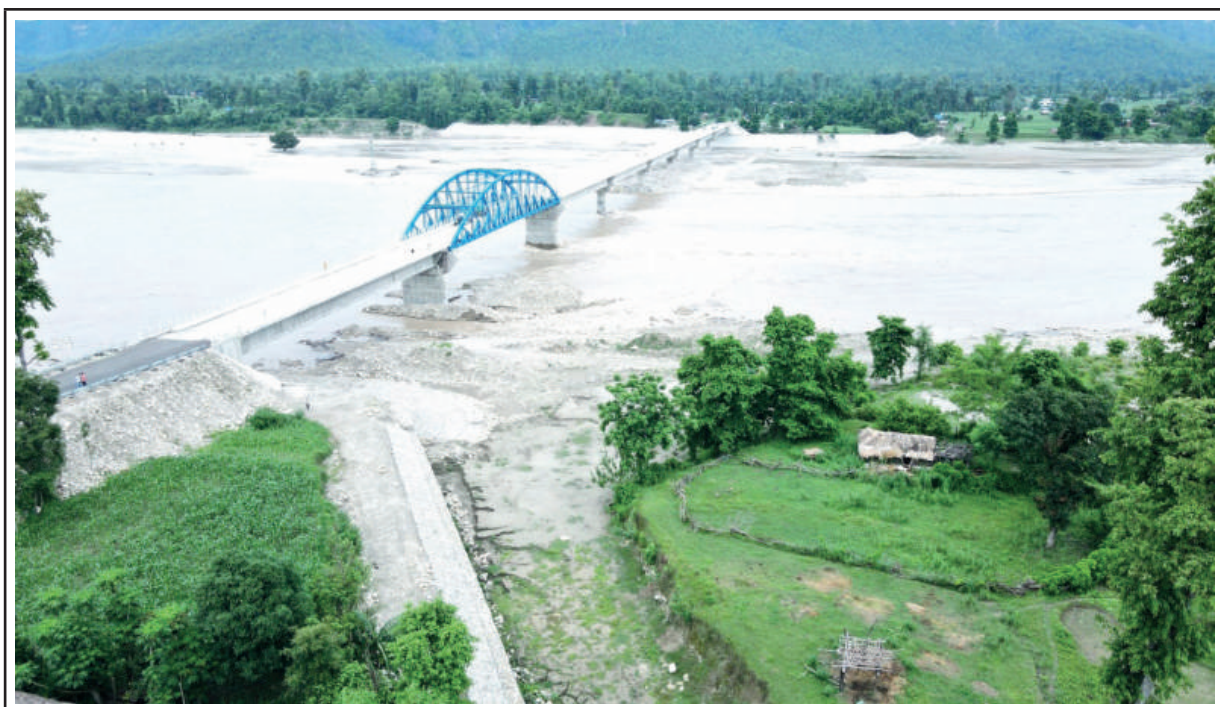
Bridge at Karnali River, Chiplegat (L=500 m)
