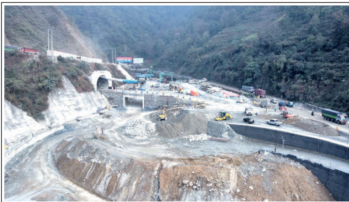
Nagdhunga Tunnel West Portal
