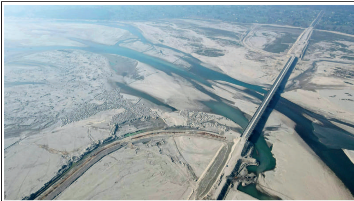
Mahakali River Bridge
