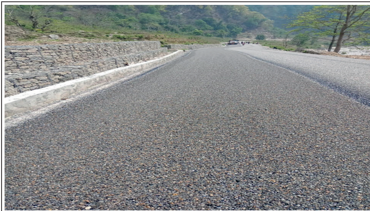
Rudhikhola- Bhainse Road, Kaski (Midhill Highway)
