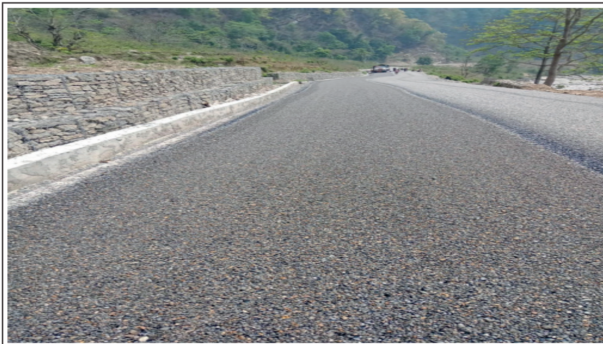
Rudhikhola- Bhainse Road, Kaski (Midhill Highway)
