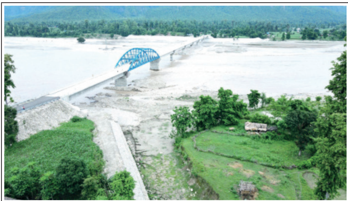
Bridge at Karnali River, Chiplegat (L=500 m)
