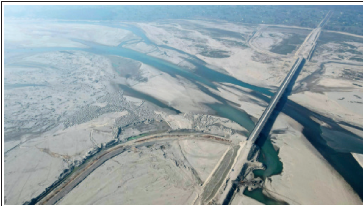
Mahakali River Bridge
