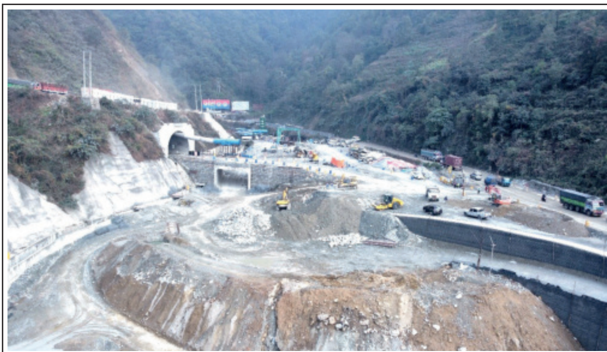
Nagdhunga Tunnel West Portal
