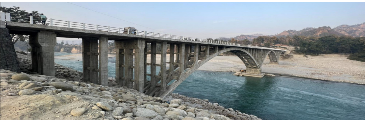
Fig. 4.5-(j) Completed Bridge
