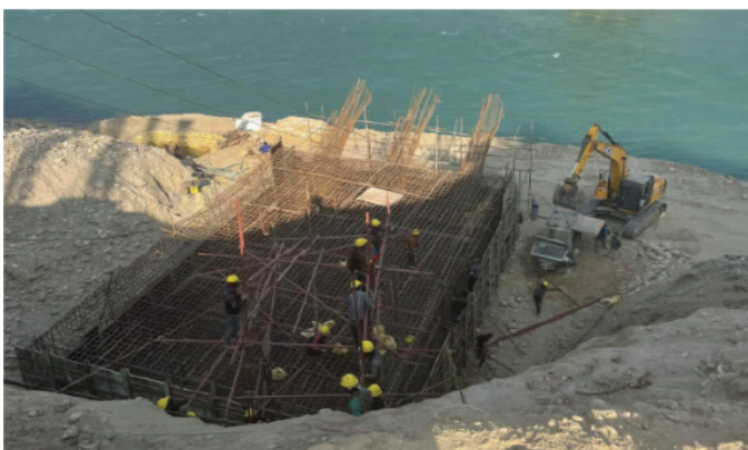
Fig. 4.4-(d) Right abutment during construction
