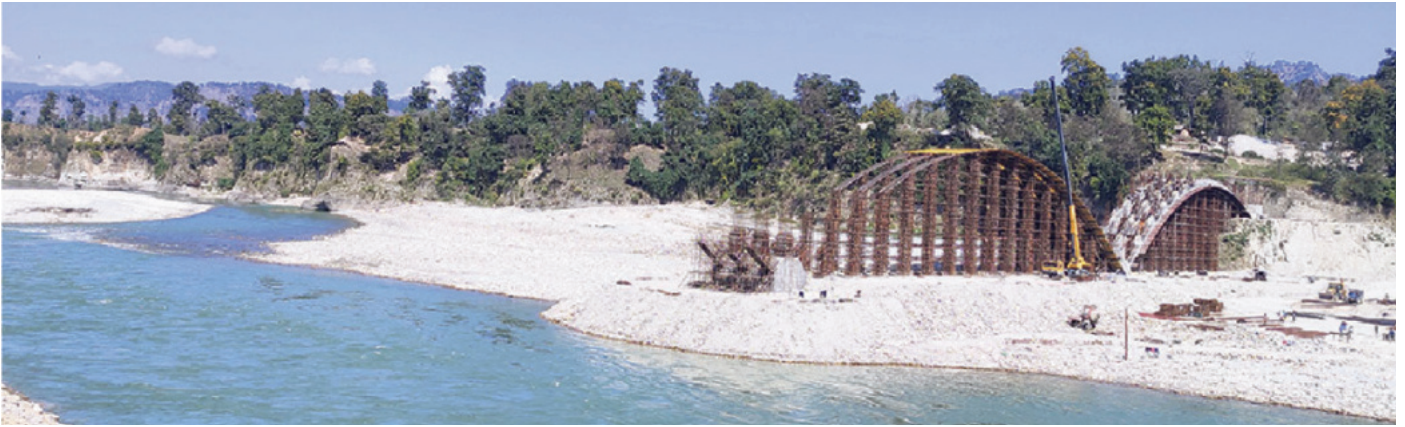
Fig. 4.4-(f) Construction of Span1 and Span2 using staging
