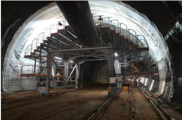
3-Setting of Geotextile and Water Proofing Membrane
