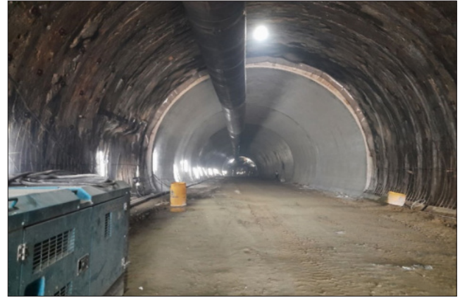
2- View of Concrete Lining
