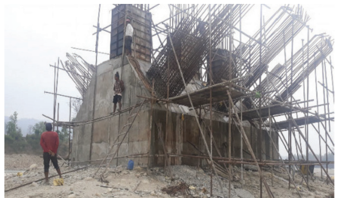
Fig. 4.4-(e) Pier during construction
