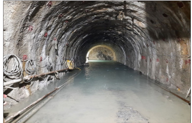
4- View of Invert Concrete
