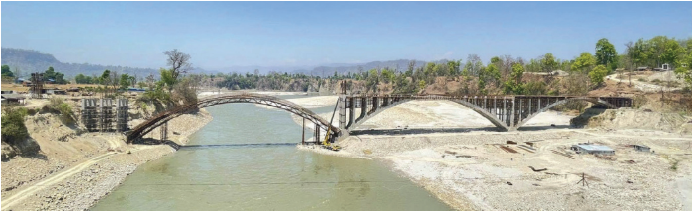
Fig. 4.4-(g) Construction of Span3 using temporary truss
