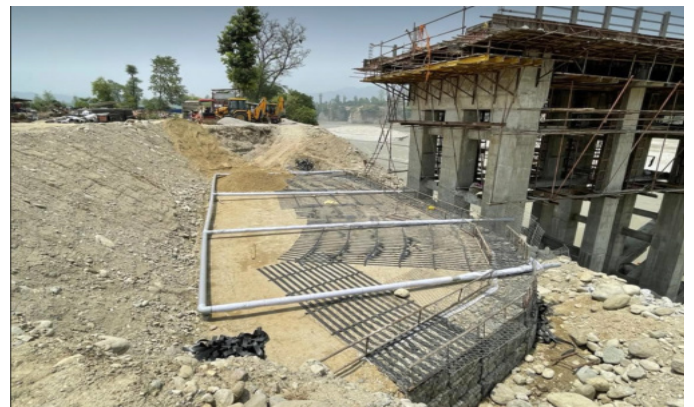
Fig. 4.5-(i) MSE wall in right abutment
