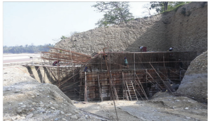
Fig. 4.4-(c) Left abutment during construction
