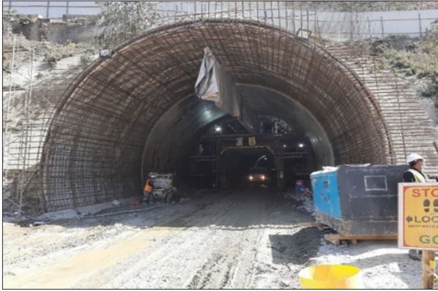
1- View of Rebar setting at Portal
