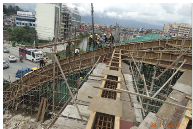
8. Preparation of concreting work of arch rib and bracing-(D/S)
