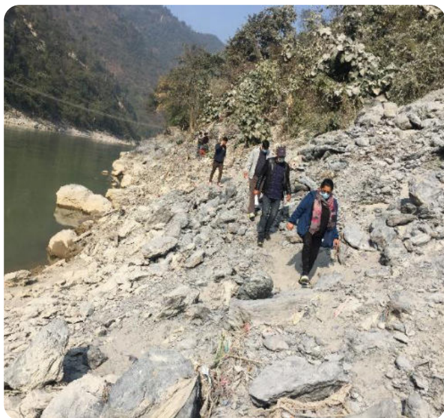
5.6 (a): Chainage 17+025 km before commencement of work
