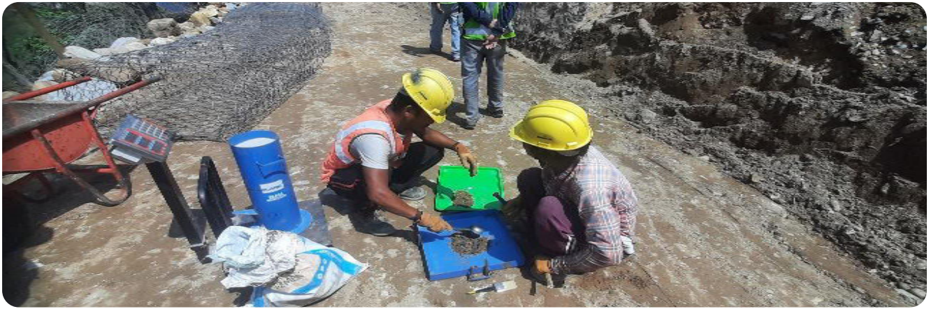
5.6 (g): Compaction test using Sand Replacement Method
