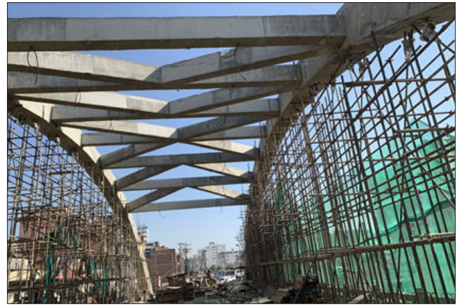
10- Arch rib and bracing after concreting (U/S)
