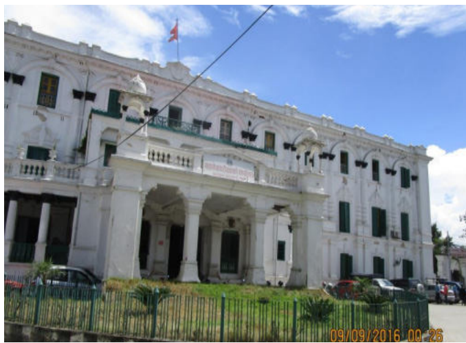
Fig. 9.1: Babar Mahal Complex before Earthquake (a) West elevation
