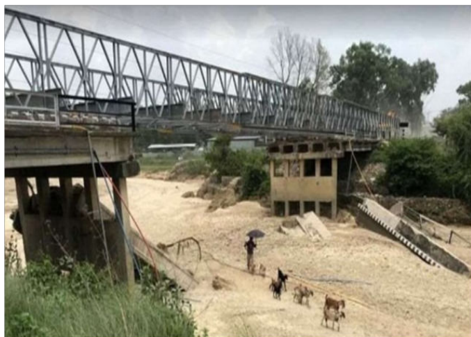
Fig. 12.3: Installed Bailey Bridge after old bridge collapse
