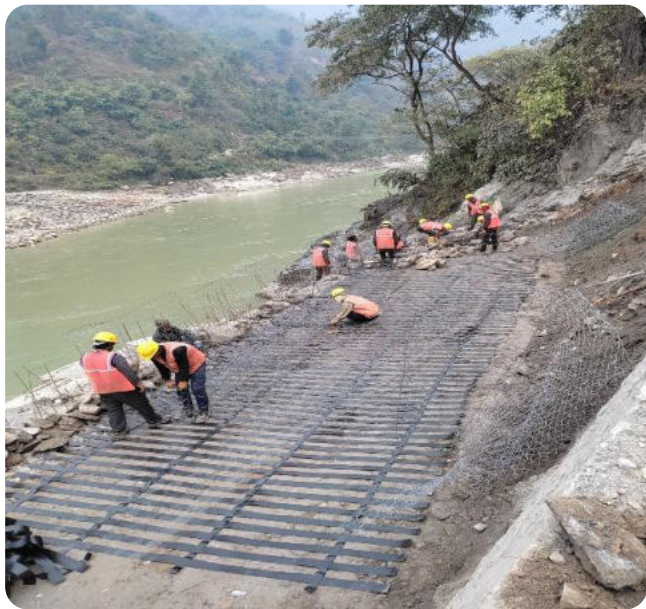
5.6 (f): Laying and placing of geogrid
