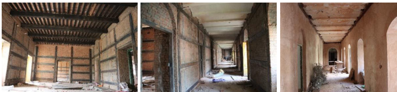
Fig. 9.8 : Inside wall Strengthening with Steel Jacketing inside wall & MS Angle for connection (a) Block A
