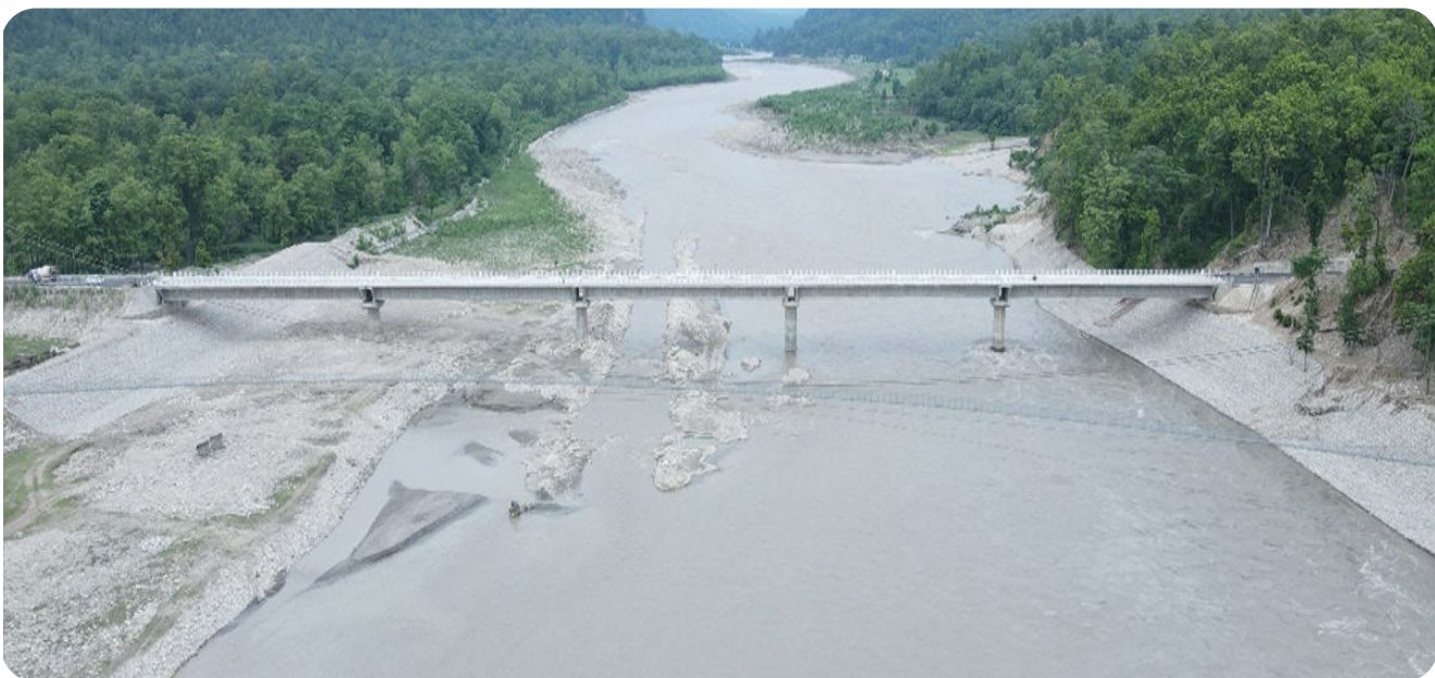
Bheri River Bridge, Khusineghat, Surkhet
