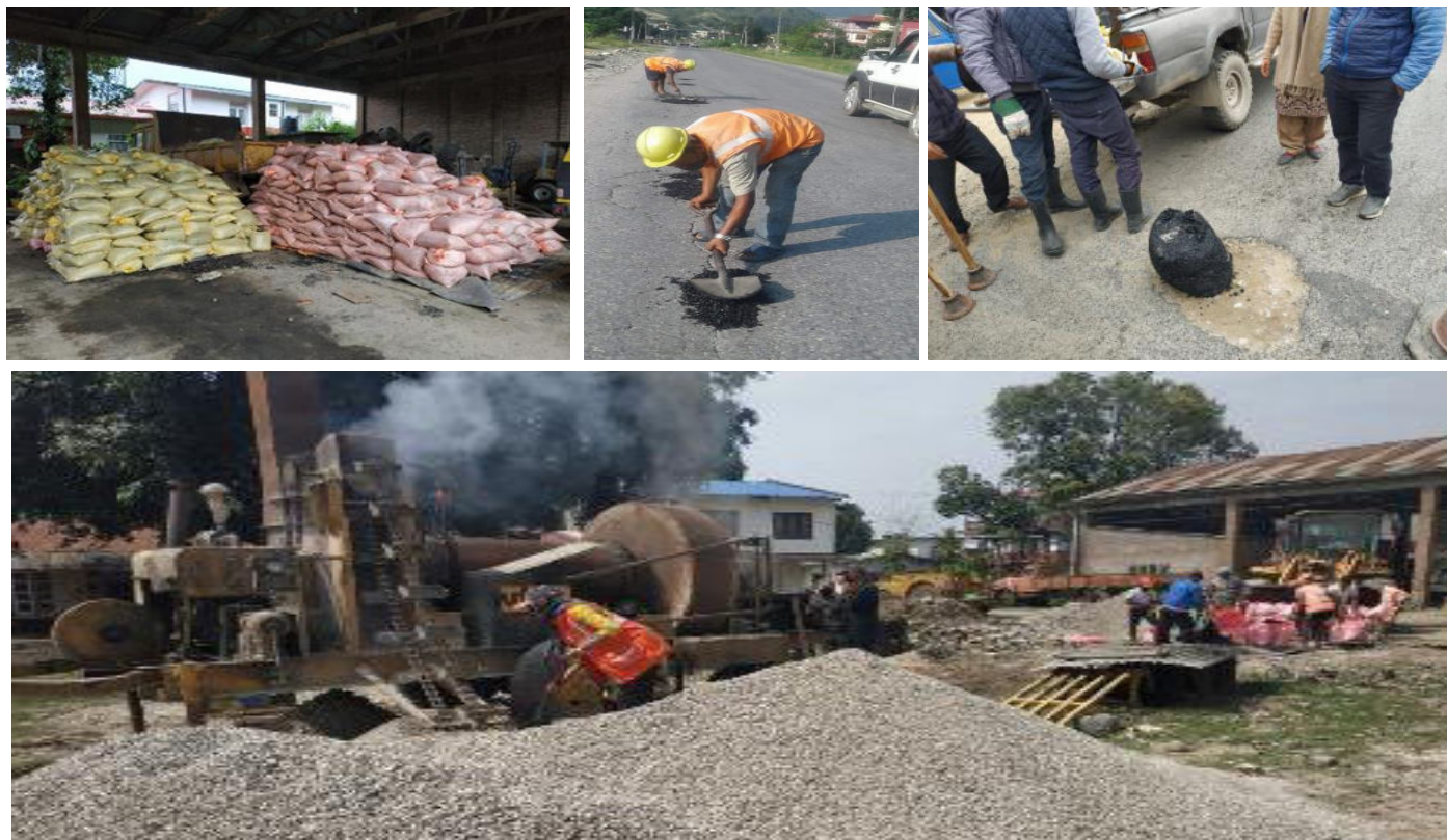
Fig. 10.4 : Photographs of materials preparation at site and laying
