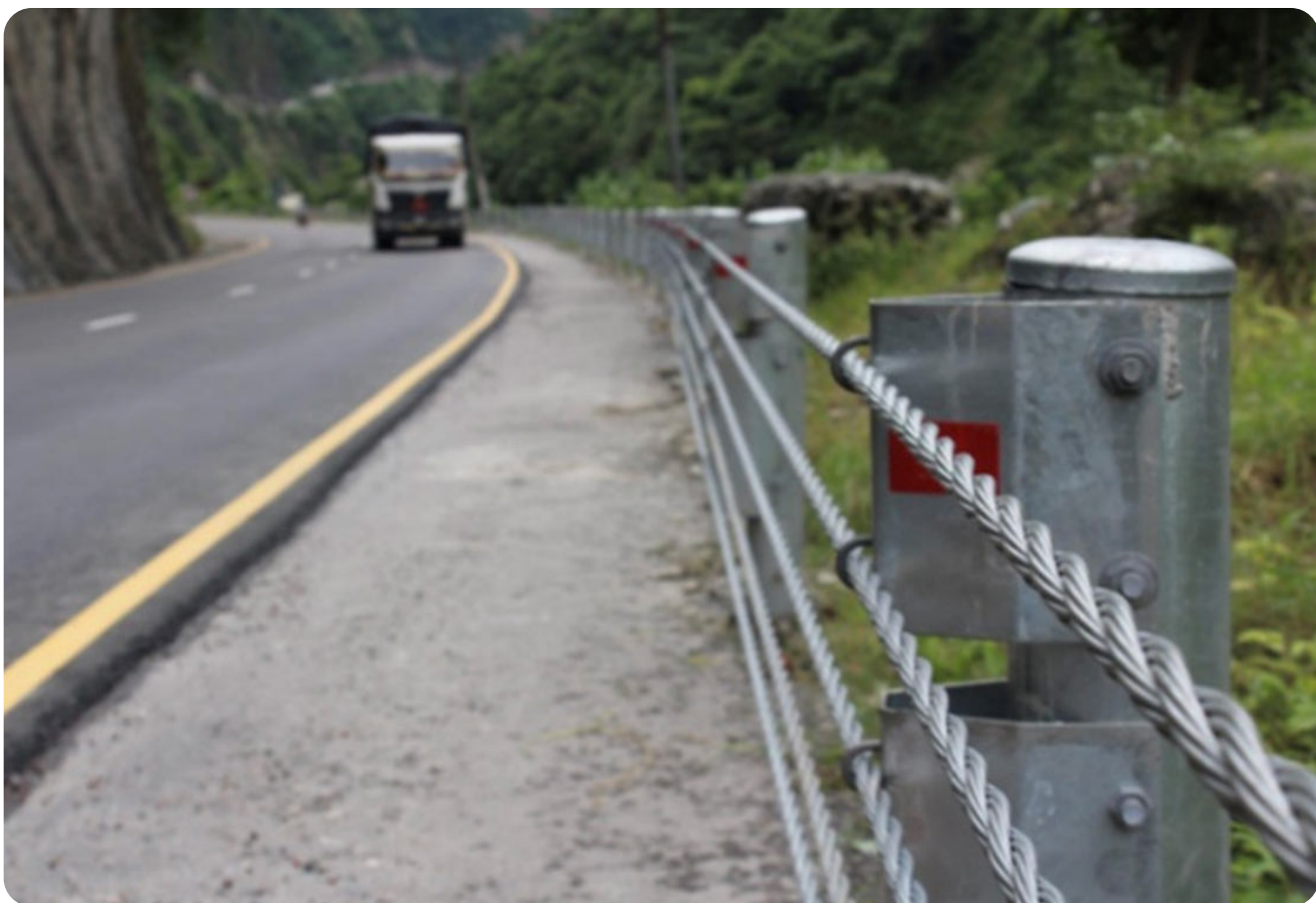
Steel-Wire-Rope-Cable-Barrier (Flexible-Guard-Rails-System) in Narayanghat-Mungling Road
