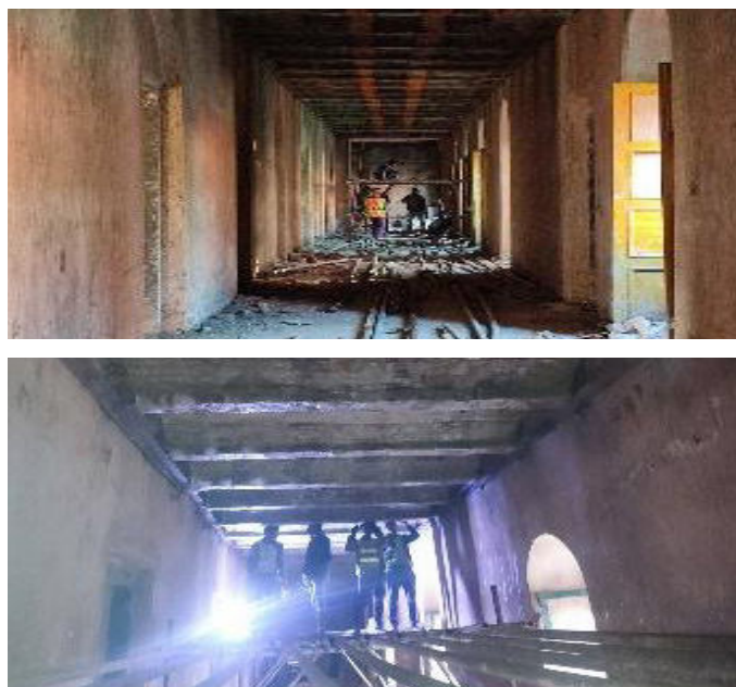
Fig. 9.6 : Jack Arch Strengthening with glass fiber
