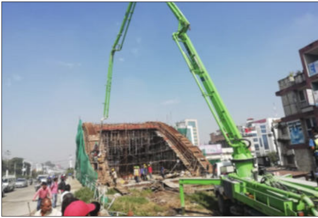
9- Concreting work of arch rib and bracing-(D/S)
