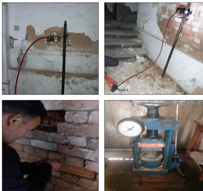
Fig. 9.4 : Typical NDT performed (a) In-situ Shear test, (b) In-situ compressive test, (c) Pocket penetrometer test, (d) Brick compressive strength test
