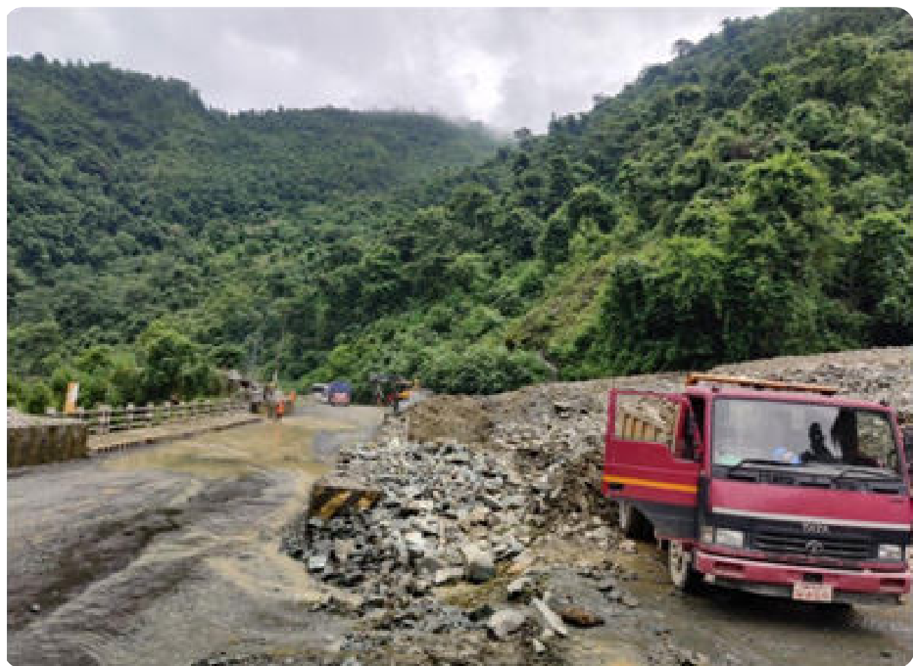
Debris flow on Narayanghat-Muglin Road at Mauri Khola Bridge
