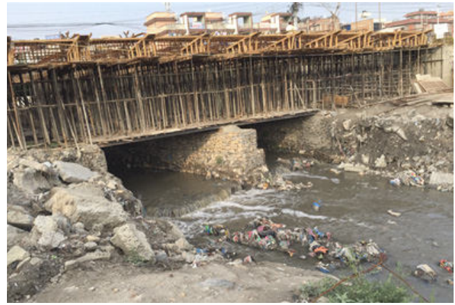
2. Temporary staging for construction of superstructure- (D/S)
