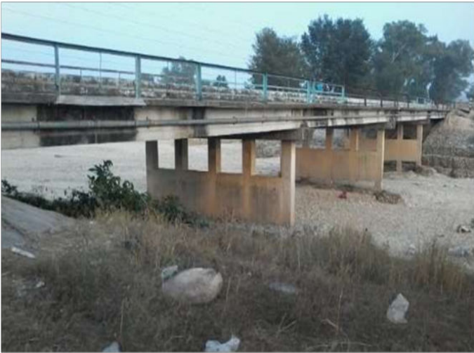
Fig. 12.1: Bridge Before collapse
