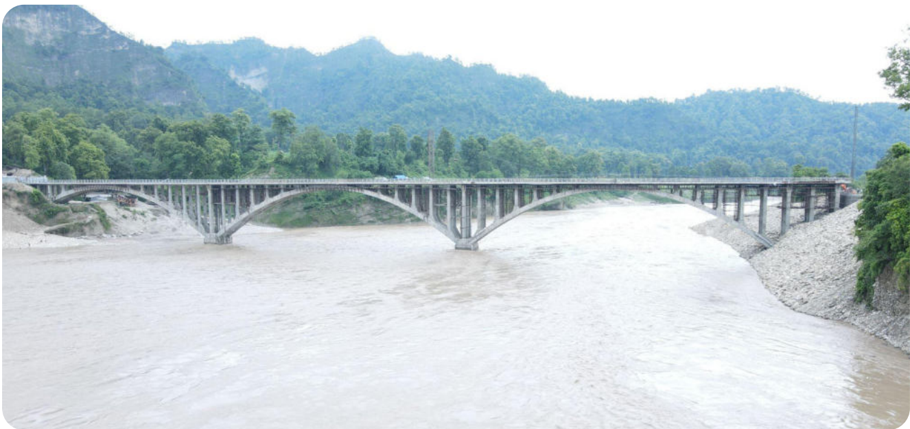
Karnali River Bridge, Kachalighat, Kuine, Surkhet
