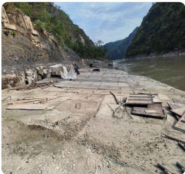
5.6 (b) : Construction of Launching Apron
