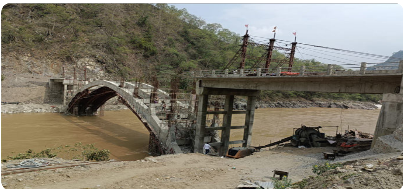
Sunkoshi River Bridge, Foxingtar
