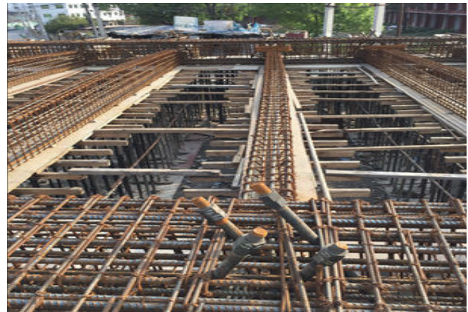
4. Construction of L and X girder-(D/S)
