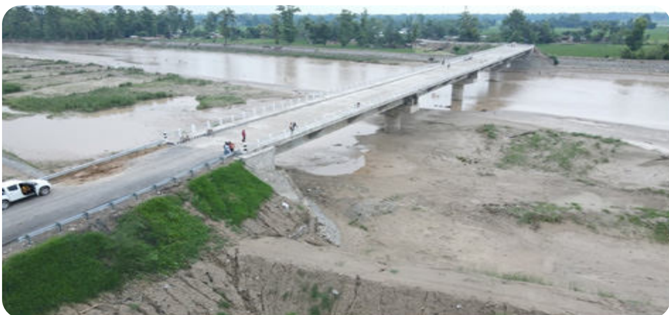
Kandra Khola Bridge, Kailali
