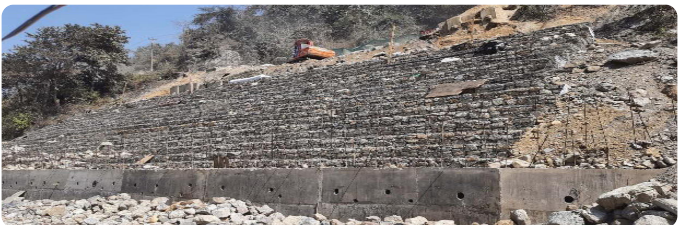
5.6 (j): Well compacted layer of geogrid and terramesh
