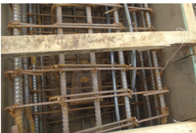
7. Details of hanger anchorage system in arch rib- (U/S)
