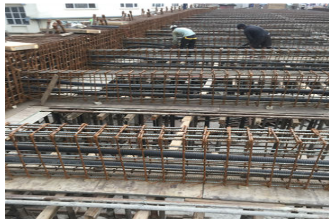
6. Duct for prestressing (post tensioning) of cross girder-(D/S)
