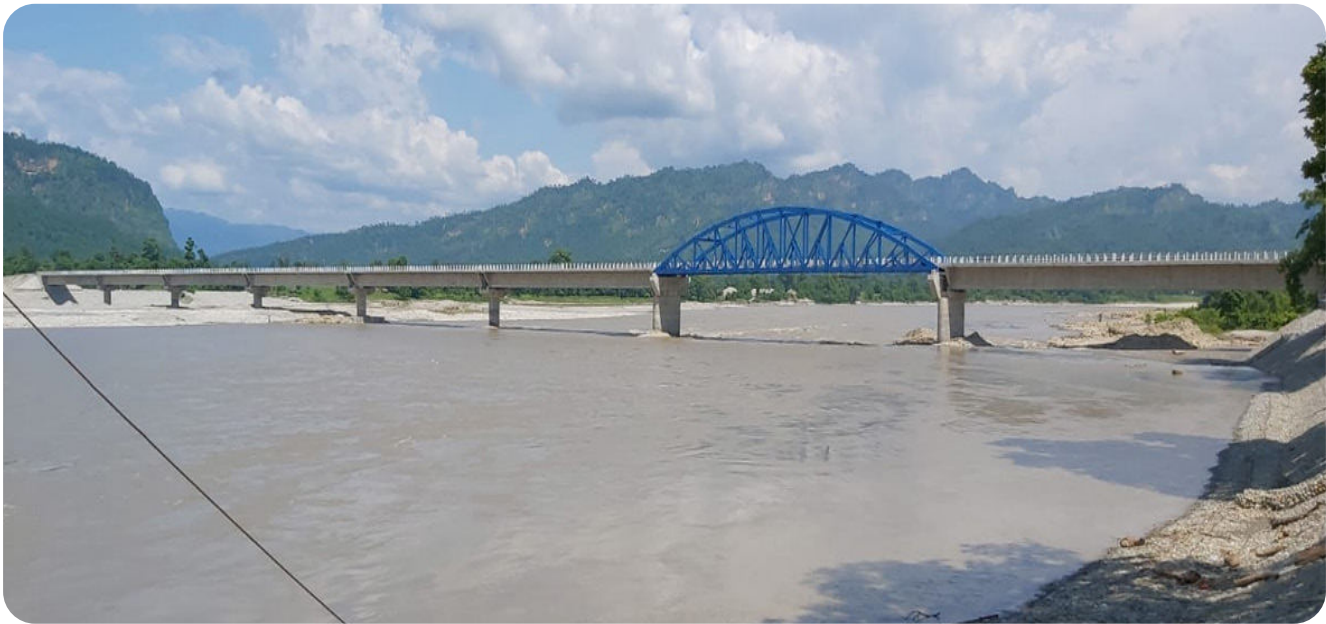
Karnali River Bridge, Chiplegat, Surkhet
