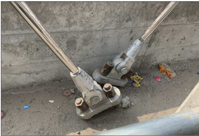
11. Hanger anchorage system –D/S
