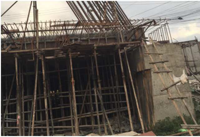
1. Construction of substructure -(D/S)
