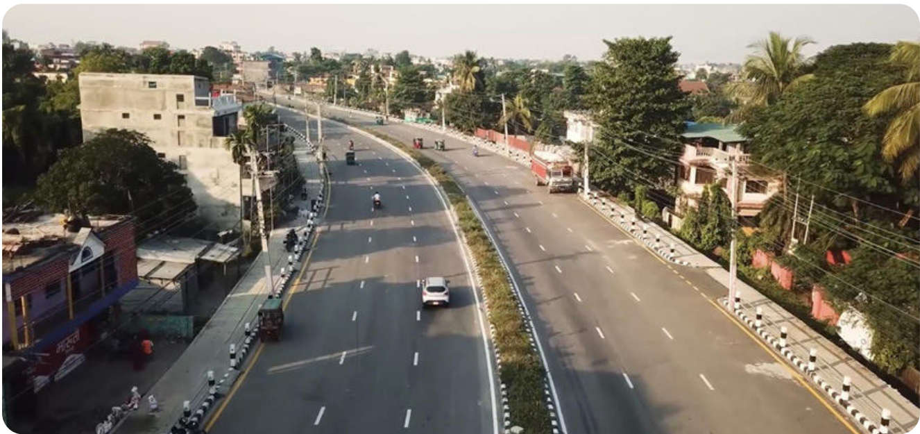
Completed Rani Nahar-Biratnagar Section (Km 3 to 6)
