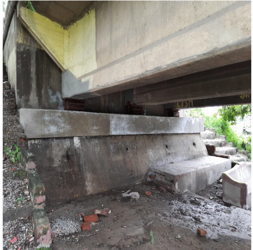
Figure 6: Repairing of abutment cap and girder with gunite material, Bakra Khola Bridge, MRM ( After Maintenance )
