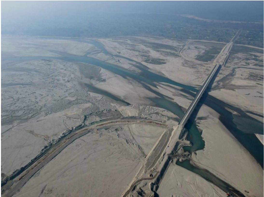
Mahakali River Bridge
