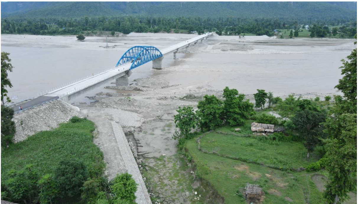
Bridge at Karnali River, Chiplegat (L=500 m)
