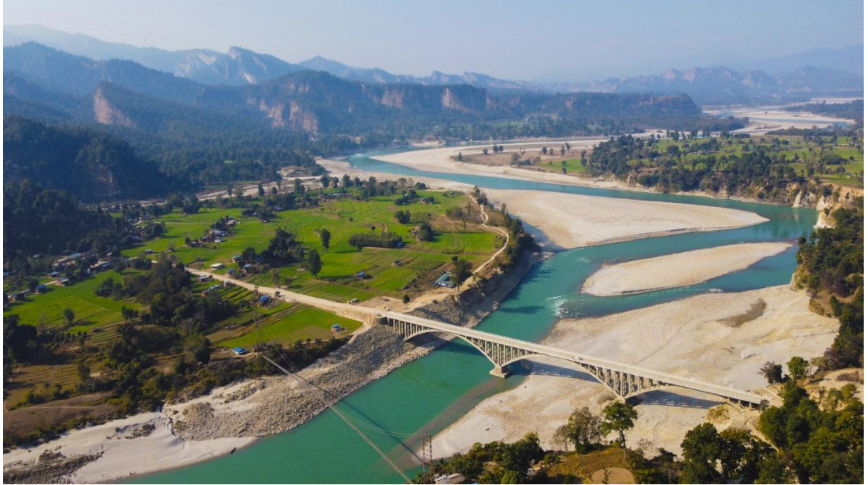
Karnali River Triple Arch Bridge, Kuine (L=300 m)
