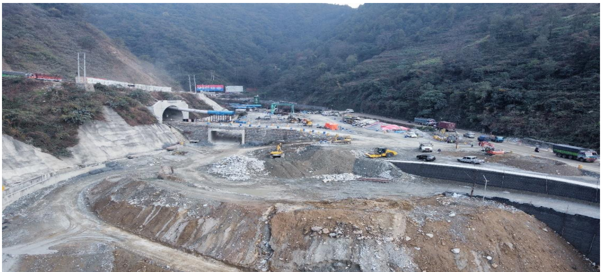
Nagdhunga Tunnel West Portal
