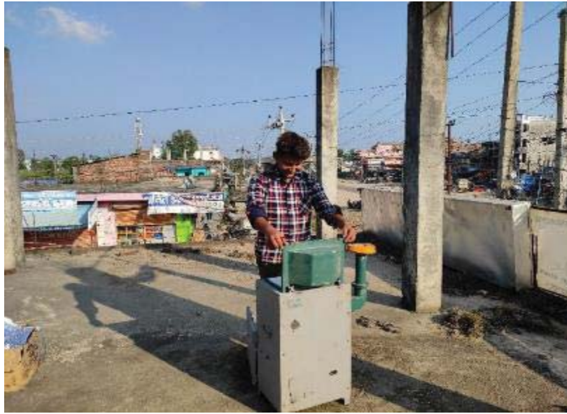
Figure 3.1: Installing High Volume Air Sampler at Dhalkebar
