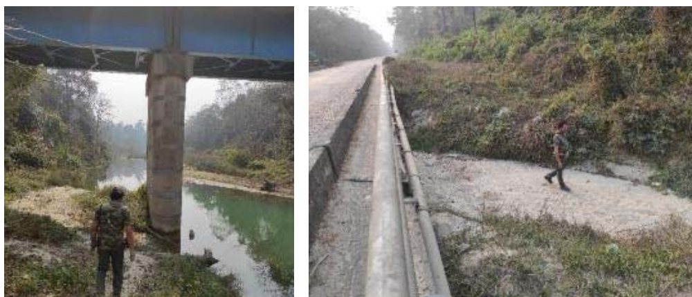
Figure 3.8: Bridge and Culvert Survey along the Project Road: a) 337+700 b)Ch 353+300
