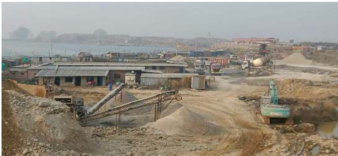
Figure 1.6: Existing Crusher Plant near Bharat Tal, Bagmati
