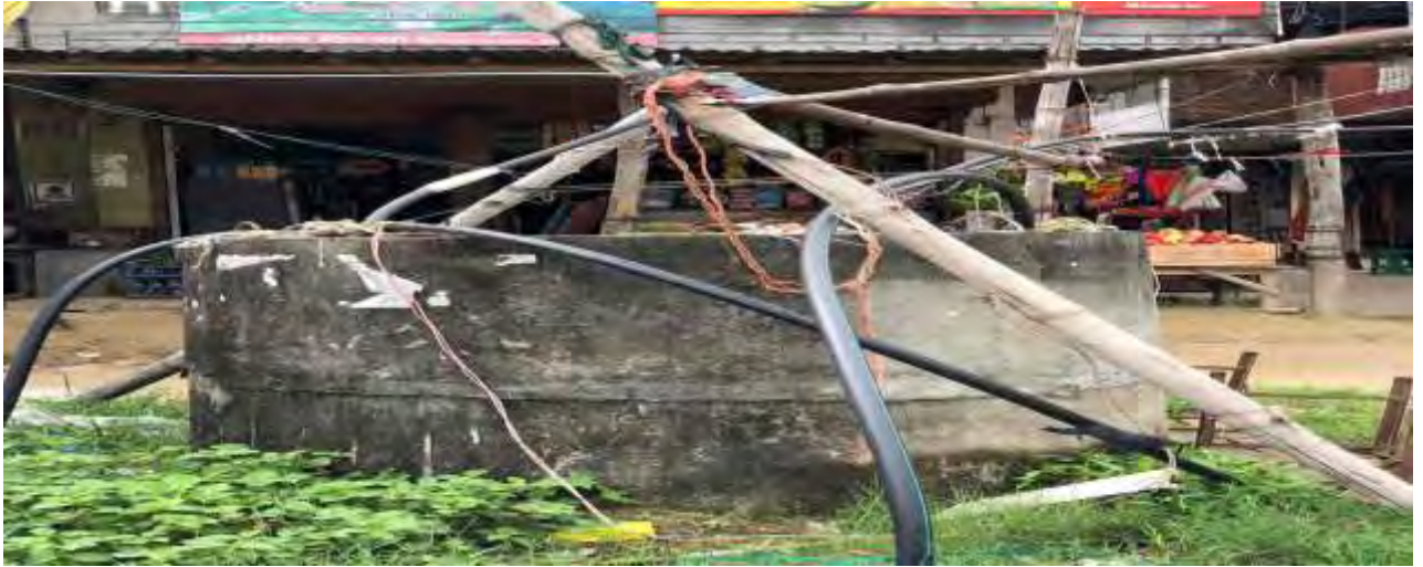
Community Structures –Well at the Edge of ROW
