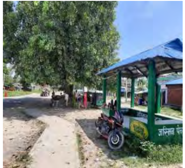
Waiting shed & Pipal Chautara at Dharapani within RoW
