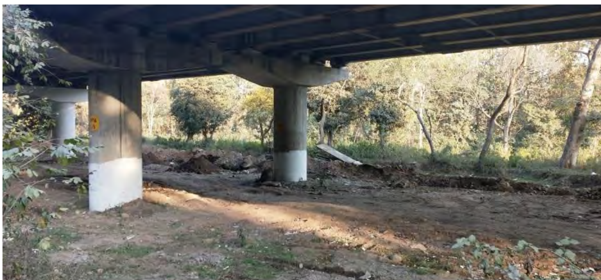
Figure 0-3: A view of the National Highway 72 underpass (6 m height) for the Elephant Chilla-Motichur corridor in Northern India.
