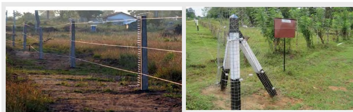
Figure 6-5: Solar Electric Fencing with Mesh Fence and Corner Supported by Jack Posts.
