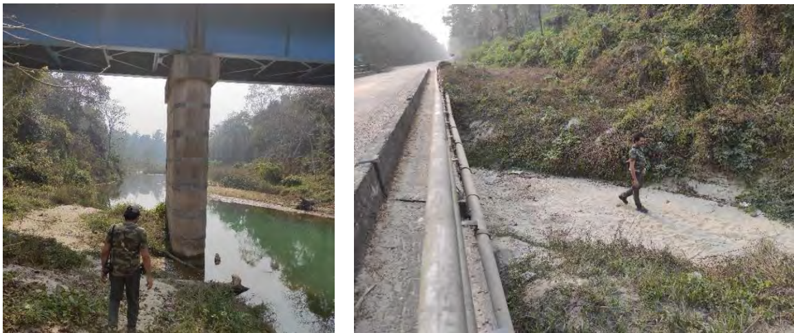
Figure 2-4: Bridge and Culvert Survey along the Project Road a) 337+700 b) Ch 353+300
