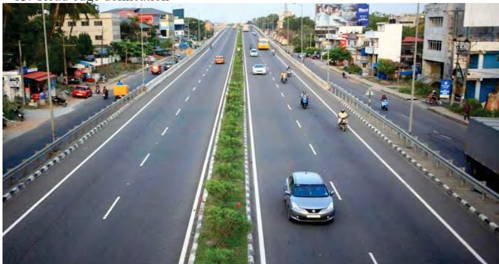
Figure 16: Typical urban section of highway
