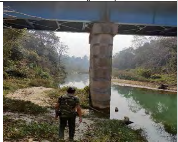
Bridge and Culvert Survey along the Project Road
