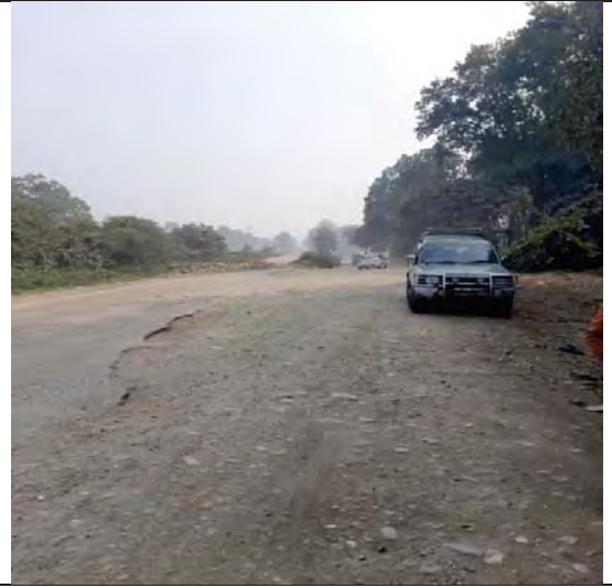
Condition of KDP Road
