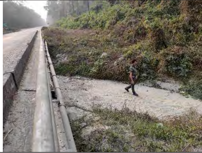
Bridge and Culvert Survey along the Project Road
