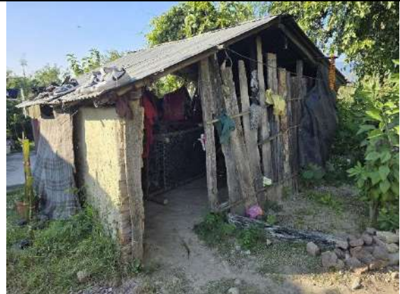
Structure no28,- Shivaraj Municipality,1, Belauti Chwok, Shed
