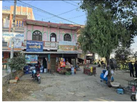
Structure no.26- Shivaraj Municipality,1, Belauti Chwok, Home
