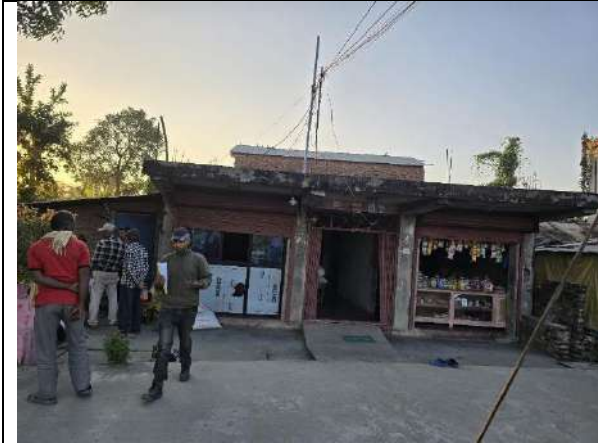
Structure no.7- Shivaraj Municipality,3, Deurali tol, Extended shed
