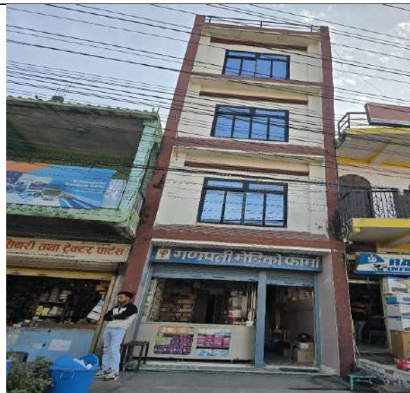
Structure no-18, Shivaraj Municipality,5, Chandrauta –Business / Residence
