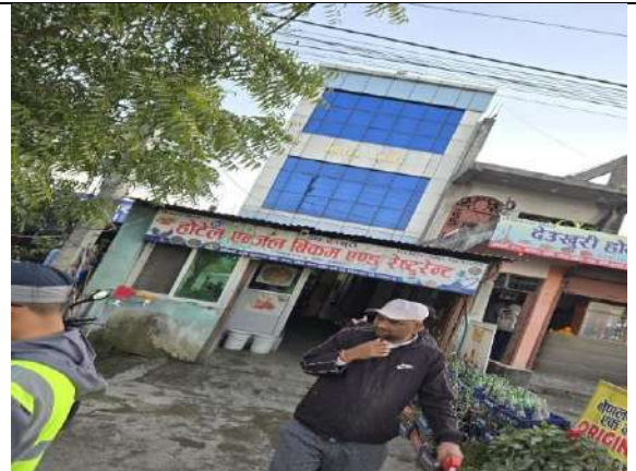
Structure no...24-. Shivaraj Municipality,5, Chandrauta –Extended room with Prifab
