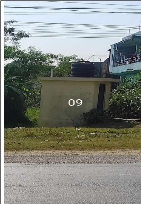
Structure no-09, Toilet, Dumara police post
