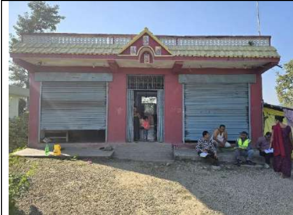
Structure no27, Shivaraj Municipality,1, Belauti Chwok, Home
