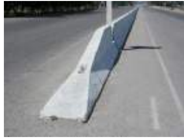
Figure 11.10: End Treatment of Concrete Barriers
