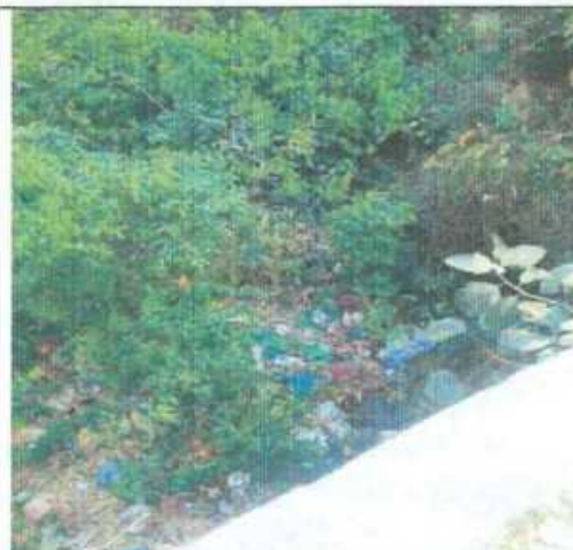
Solid waste dumps in the Culvert area (CH 649+400)
