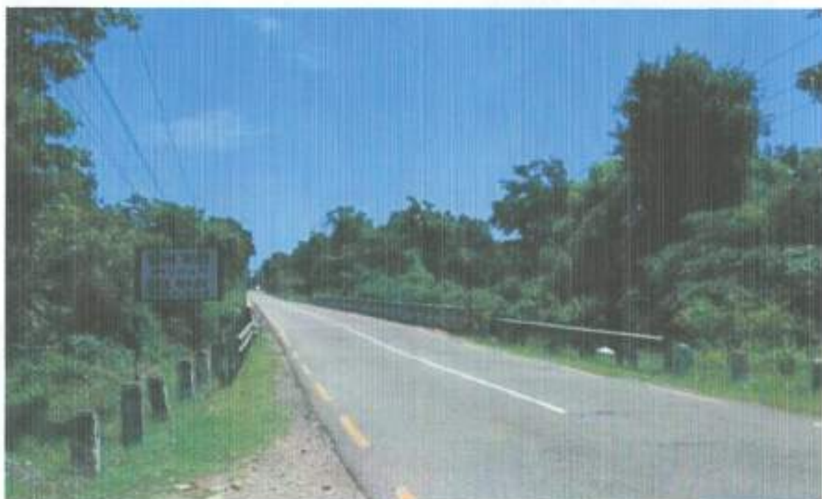
Figure 3-16: Photo showing Belnadi bridge
