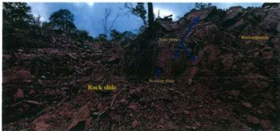
Figure.6: Photograph basement rock exposed in the landslide area
