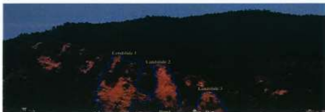
Figure 3: Butwal Landslide delineation observed at chainage 591+300 to 591+400
