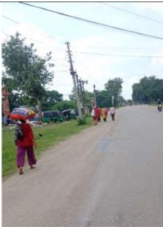
Figure 80 Absence of Footpath at Pipra
