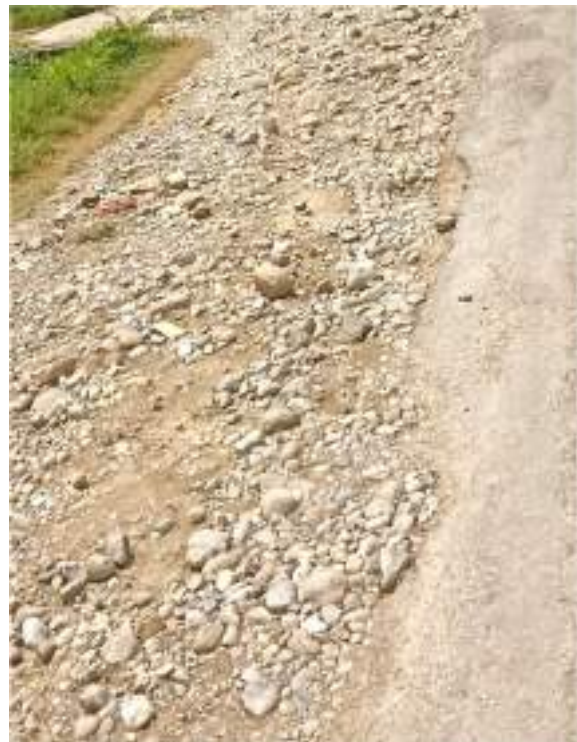
Figure 69 Exposed Base at Kalauni
