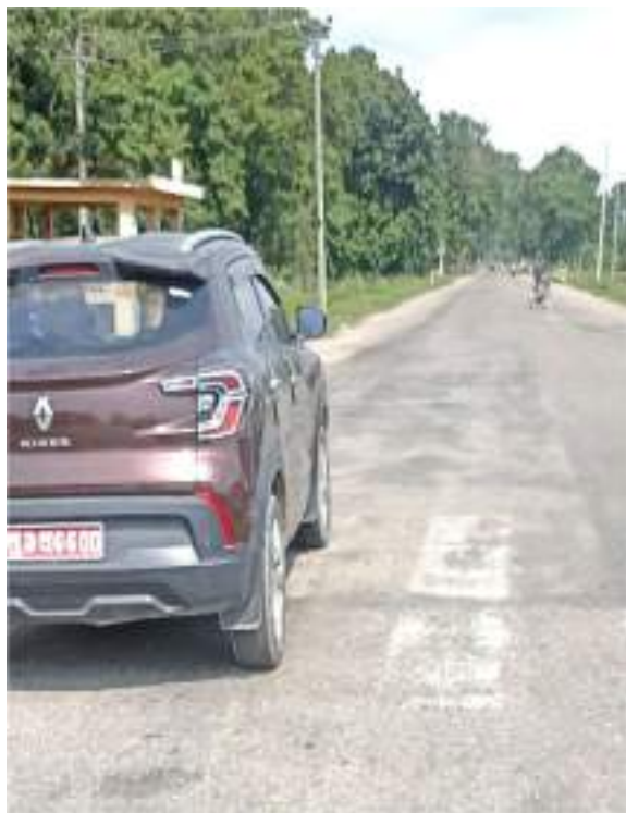
Figure 84 Unclear zebra crossing lines at Farline Jungle
