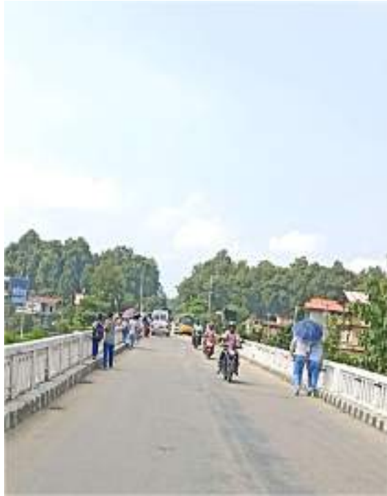
Figure 82 Absence of footpath at Saljhandi bridge
