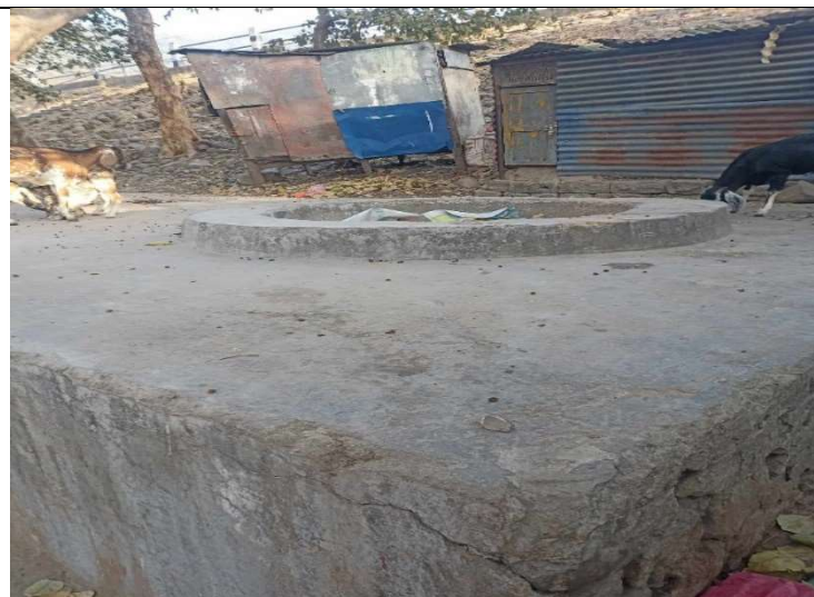
Well located at the Bridge Site
