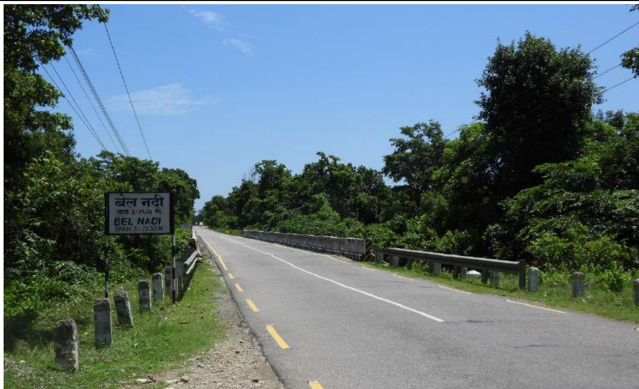
Photo Plate 3- 5: Photo showing Belnadi bridge (Source Field survey: 2024)
