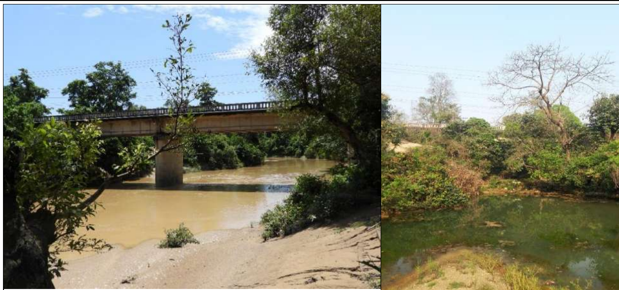
Photo Plate 2-3: Belnadi bridge and water body below Jwai khola bridge use by wildlife for drinking (Source: Field survey, 2024)
