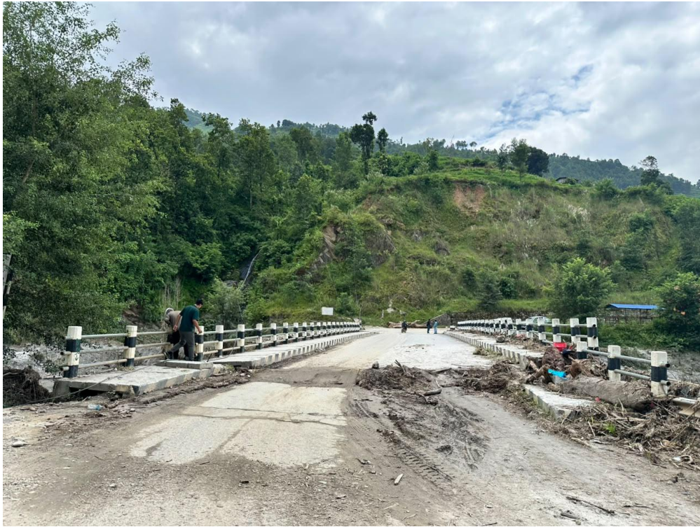
Figure 14 Road surface on the bridge showing mud and debris deposits
