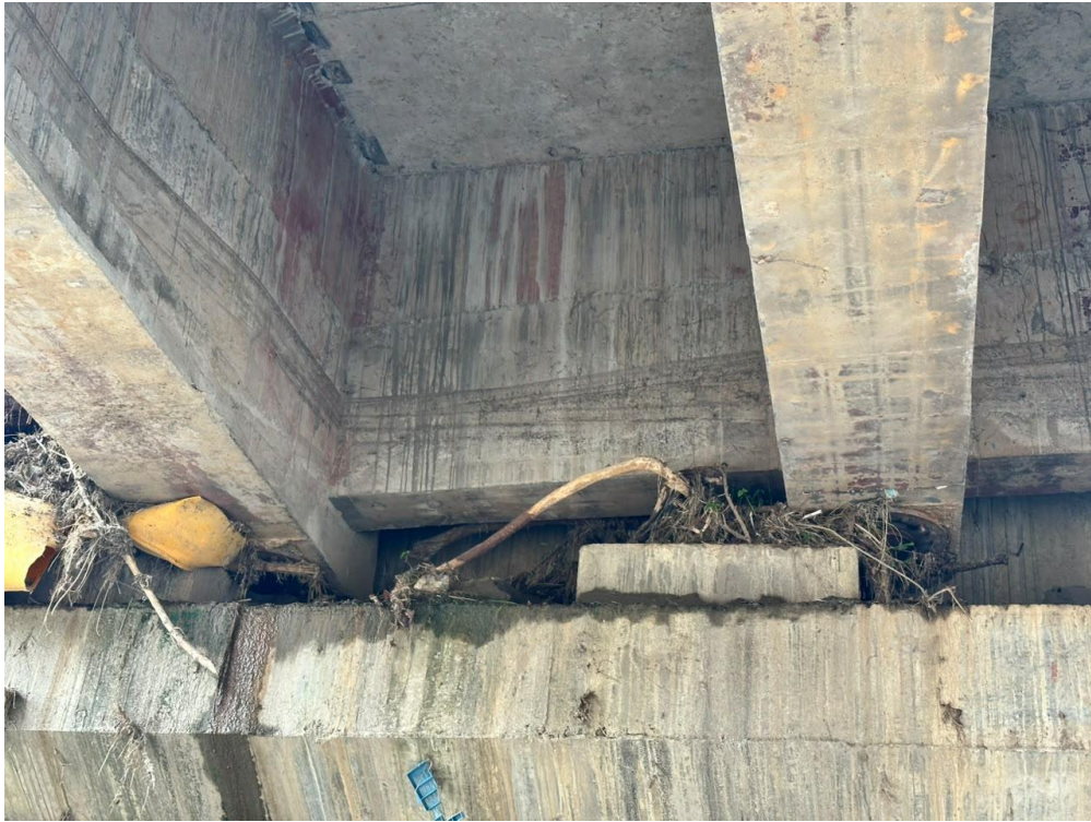
Figure 8 Underside of bridge showing debris
