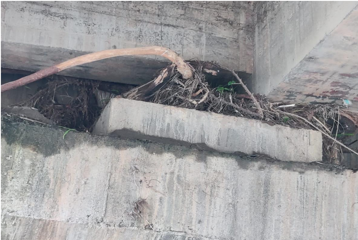
Figure 1 Close-up view of debris accumulation under the bridge girders
