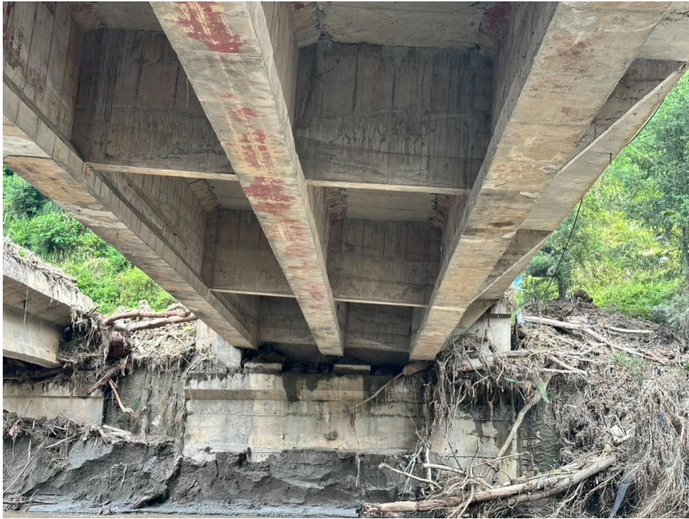
Figure 10 View showing shifting and tilting of Bridge deck and position of Girders
