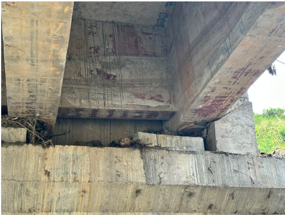
Figure 10 View showing shifting and tilting of Bridge deck and position of Girders
