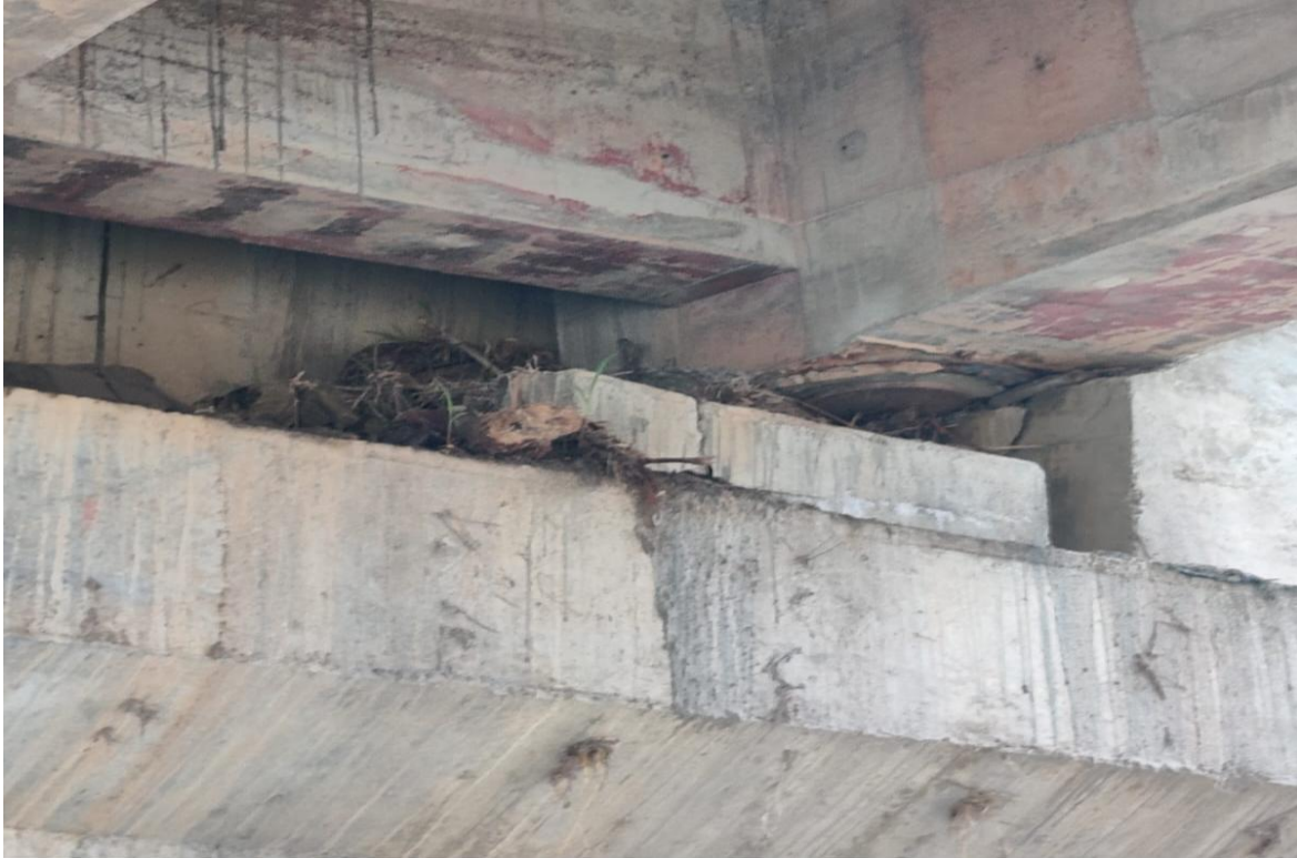
Figure 1 Close-up view of debris accumulation under the bridge girders
