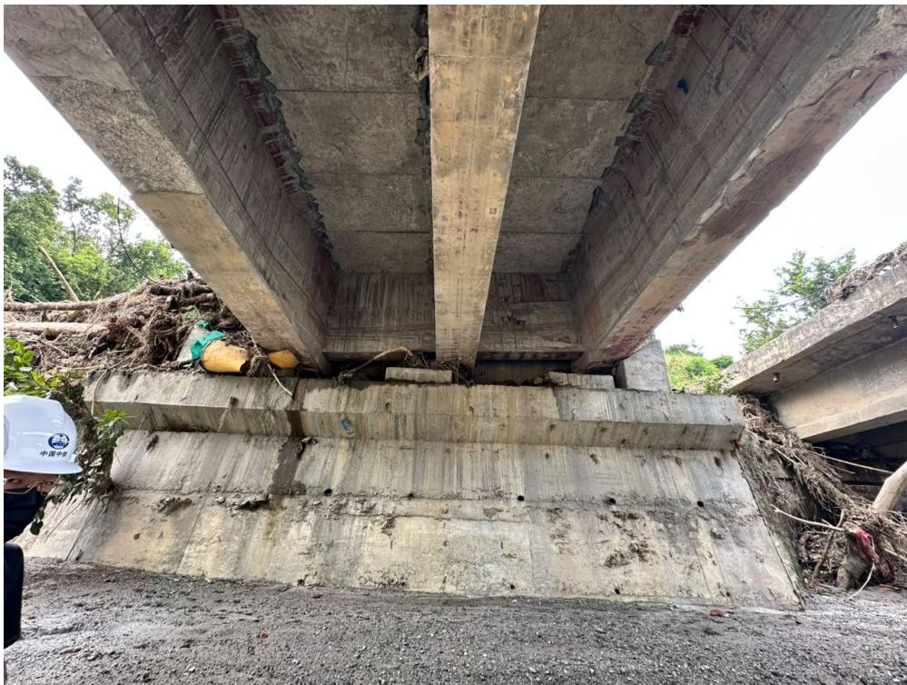
Figure 8 Underside of bridge showing debris
